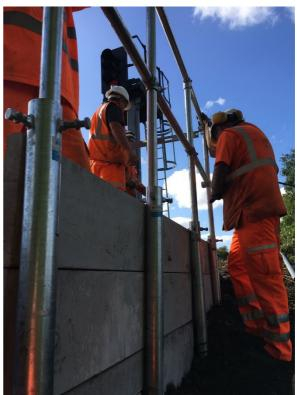
A 4-man team installed the required 12 No screws, fixing both the gravel boards and handrail over a single 8-hr shift.
